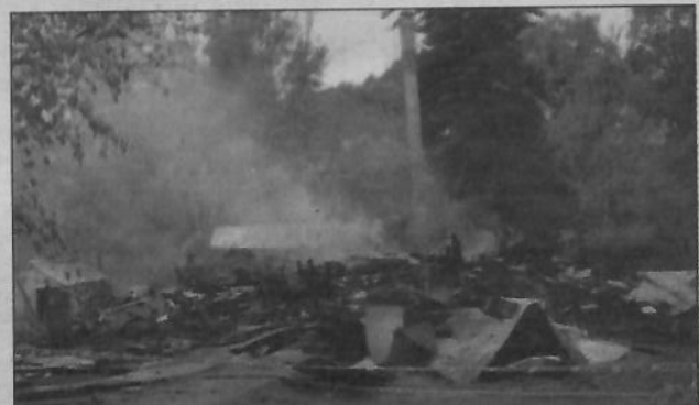
The chimney was all that was left standing from a fire that consumed a residence on County Road 7 Monday evening. The cause of the fire is under investigation by the Colorado Bureau of Investigation.
